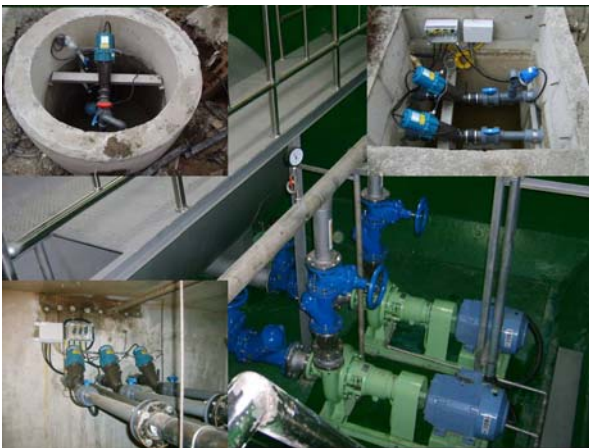
Underground station, collection chambers has 1 to 3 vacuum valves installed due to the flow.
