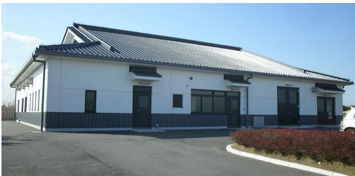
Vacuum- Station with water purification plant
